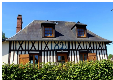
Maison, façade est. Phot. Gaëlle Pottier IVR28_20197606337NUCA
